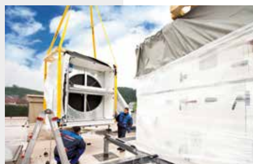
Delivery and installation of a weatherproof X-CUBE
